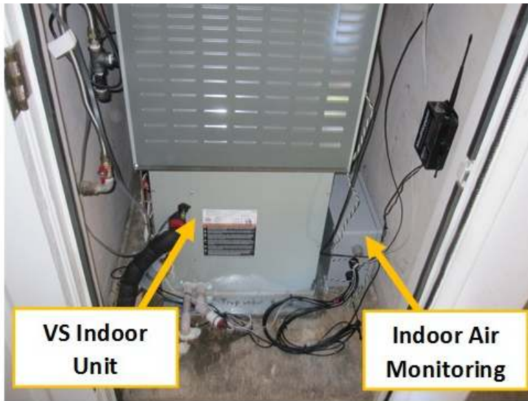
FIGURE 17. INDOOR UNIT AND INDOOR AIR MONITORING AT FIELD SITE 3
