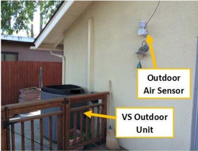
FIGURE 7. OUTDOOR UNIT AND OUTDOOR TEMPERATURE SENSOR AT FIELD SITE 1
