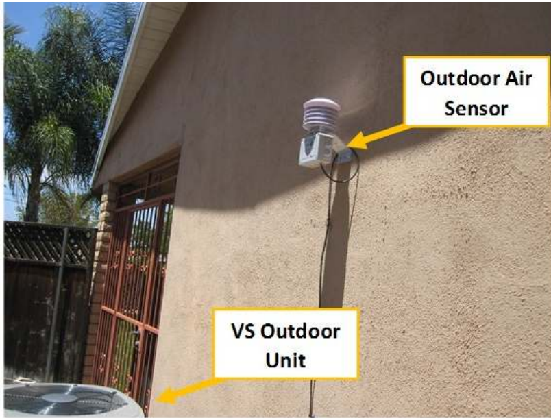
FIGURE 16. OUTDOOR UNIT AND OUTDOOR TEMPERATURE SENSOR AT FIELD SITE 3
