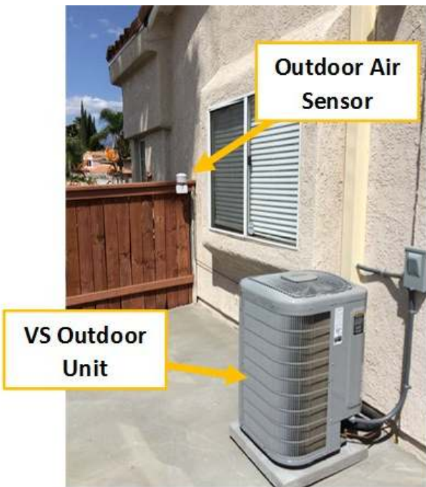
FIGURE 12. OUTDOOR UNIT AND OUTDOOR TEMPERATURE SENSOR AT FIELD SITE 2
