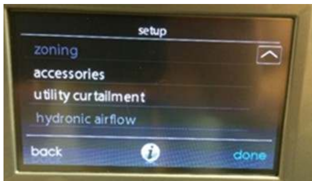
FIGURE 36. LABORATORY DR ASSESSMENT: DR SETUP ON UNIT CONTROLLER – VC SYSTEM 2
