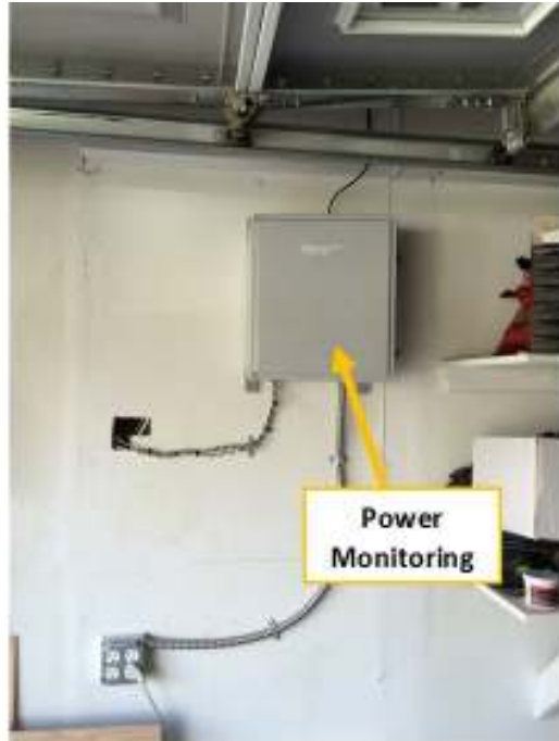
FIGURE 11. POWER MONITORING AT FIELD SITE 2
