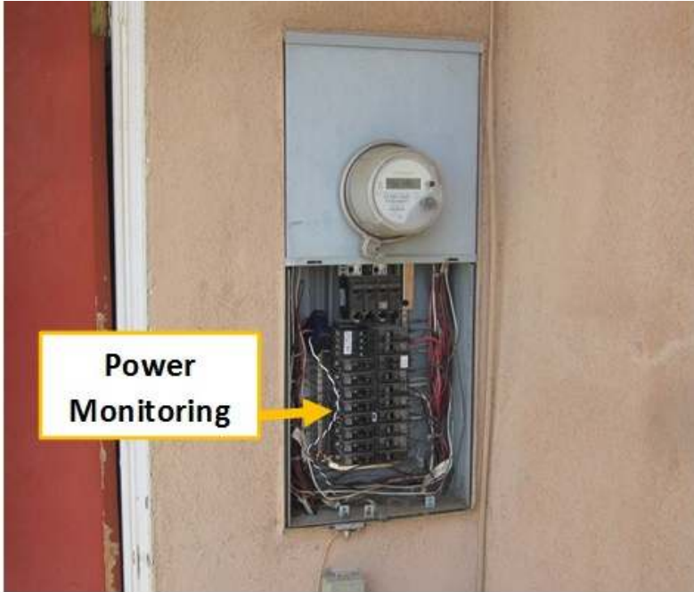
FIGURE 15. BREAKER PANEL AND POWER MONITORING AT FIELD SITE 3
