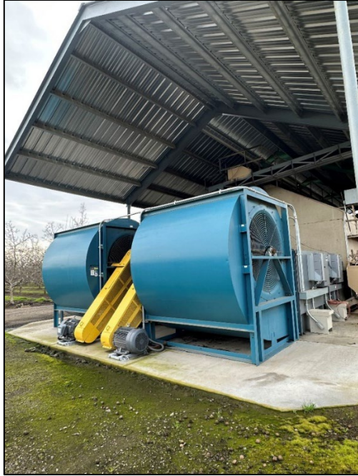
Figure 4: Natural gas burners and fan units
