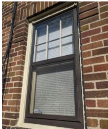
Figure 3. Storm Window Add-On [11]
