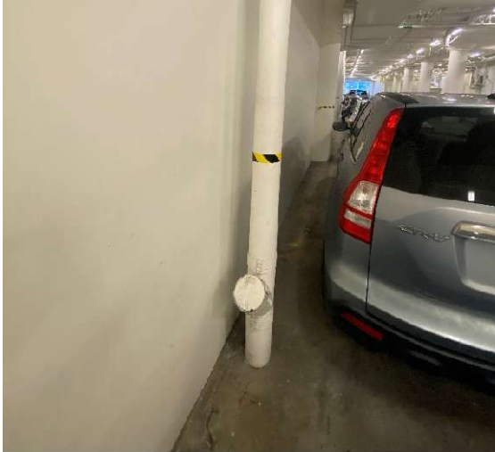
Figure 26: One of four sewer risers in Commercial Office Building A parking garage.
