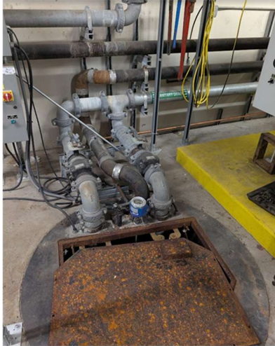
Figure 24: Hospital B sanitary pipe and tank.
