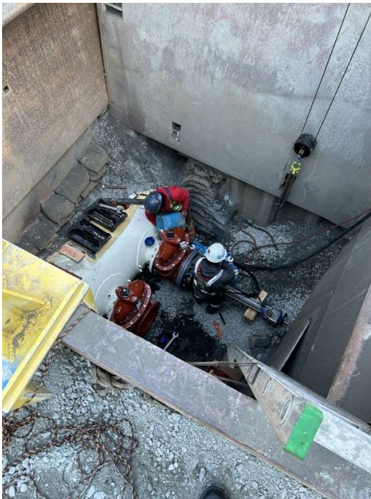
Figure 22: Hot tapping sewer main.
