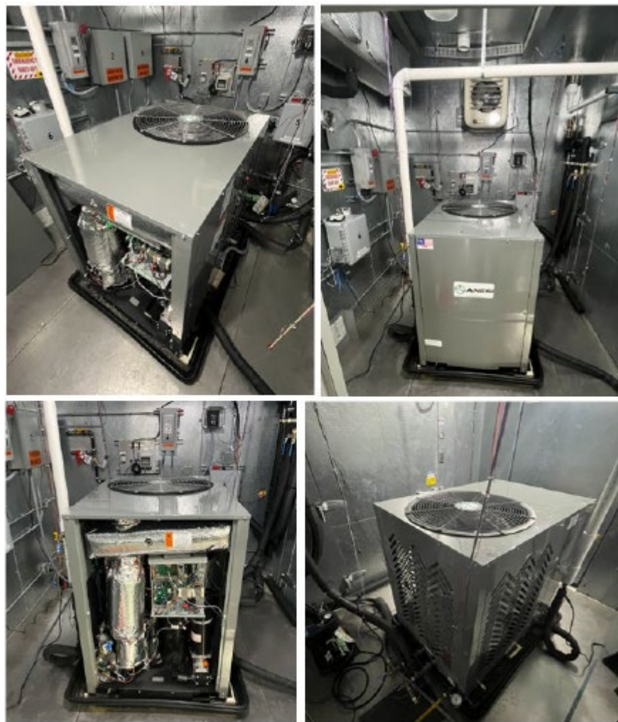
Figure 2: GAHP Installation Pictures.
