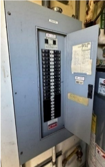
Figure 64: 100 A 208 V single phase electrical panel for sites #5 and #6.
