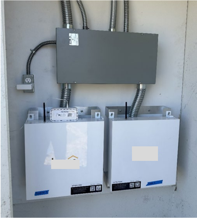
Figure 69: Completed installation of both smart subpanels at sites #5 and #6.
