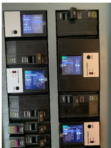
Figure 103: Smart Breakers installed at site #9
