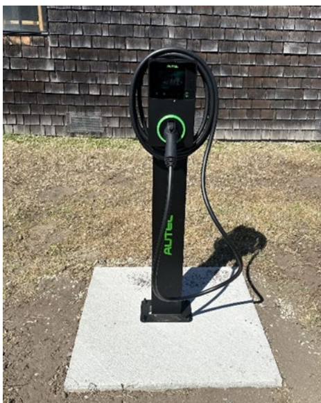
Figure 39: A Level 2 EV Charger installed at site #2.
