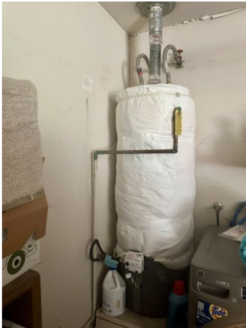
Figure 60: Existing gas fired water heater at site #4.
