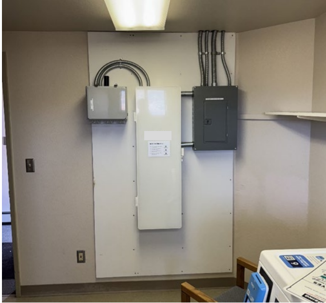
Figure 41: Post-installation of smart panel infrastructure at site #2.
