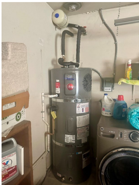
Figure 61: HPWH installed at site #4
