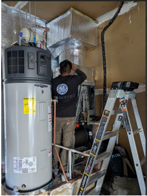
Figure 30: HPWH installed at site #1.
