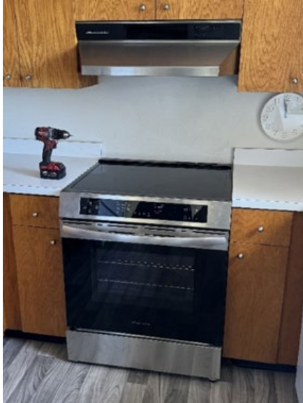
Figure 66: 50 A inductive cooktop installed at site #5.
