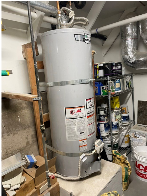
Figure 53: Existing gas fired water heater at site #3.
