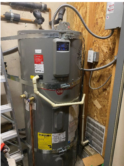
Figure 101: HPWH installed at site #9.
