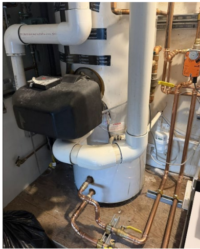
Figure 93: Space and DHW HPWH installed at site #8.
