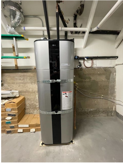
Figure 54: HPWH installed at site #3.
