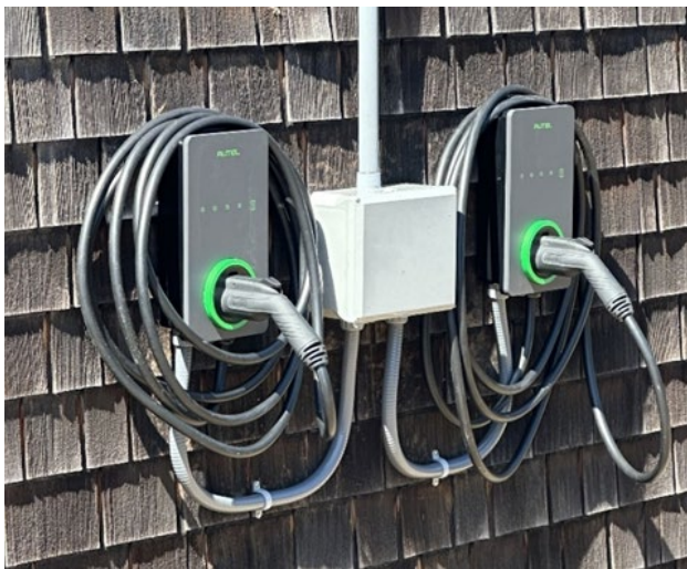
Figure 67: Both 32 A Level 2 EV charger installed at sites #5 and #6.
