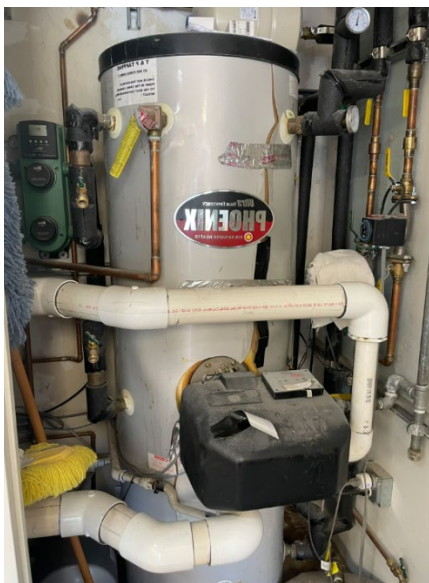
Figure 91: Existing gas fired water heater at site #8.
