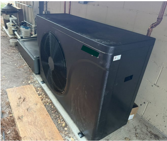
Figure 92: Space and DHW HPWH installed at site #8.
