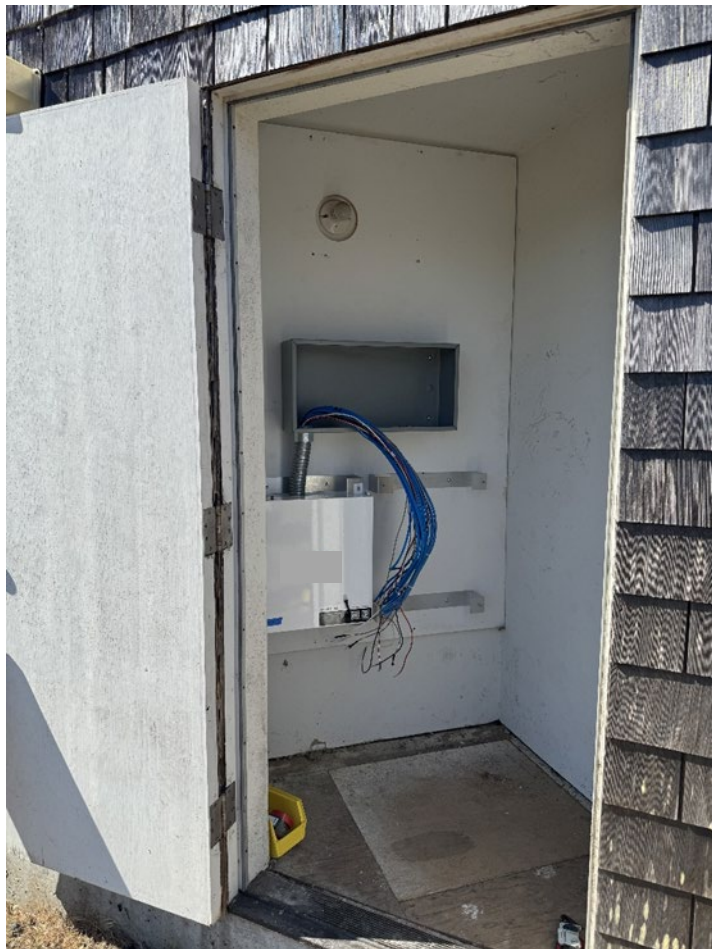
Figure 68: Smart subpanel installation at the duplex.
