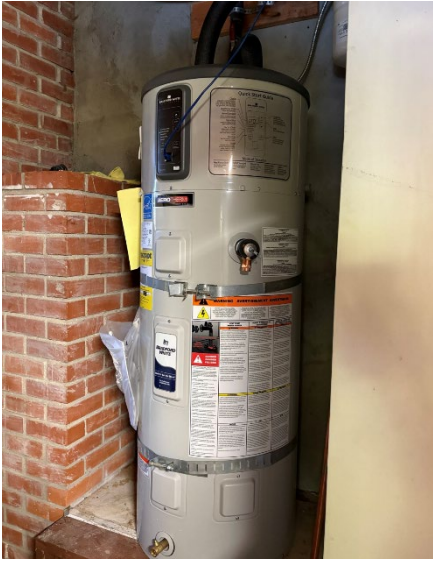
Figure 86: HPWH installed at site #7.
