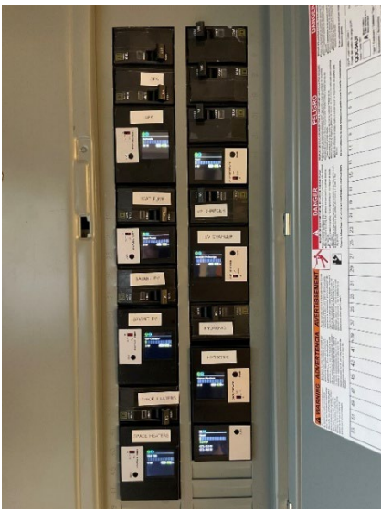
Figure 94: Smart Breakers installed at site #8.
