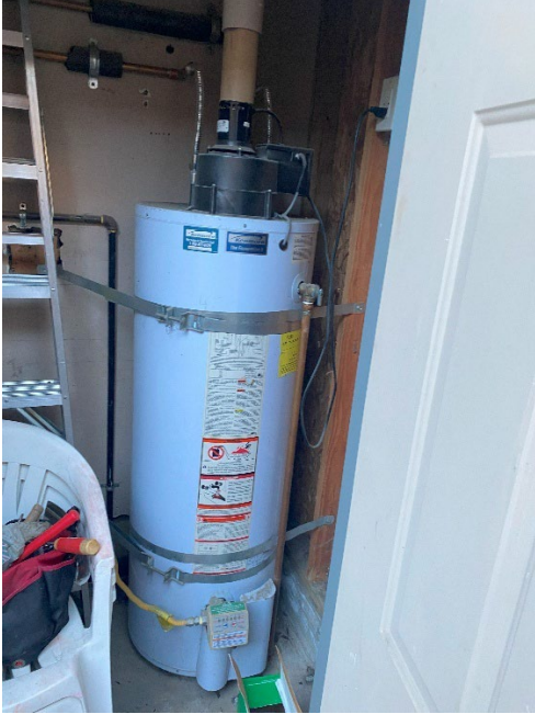
Figure 98: Existing gas fired water heater at site #9.
