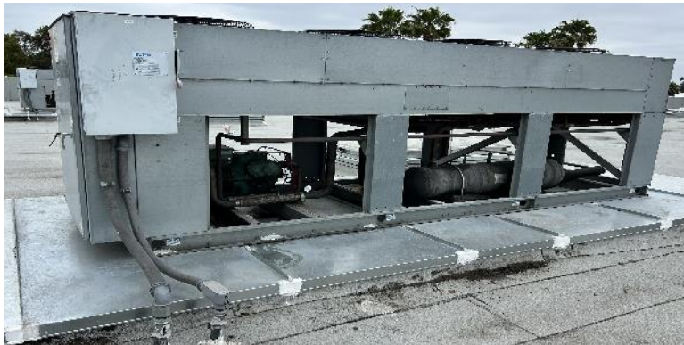
Figure 7: CU4 condensing unit.
