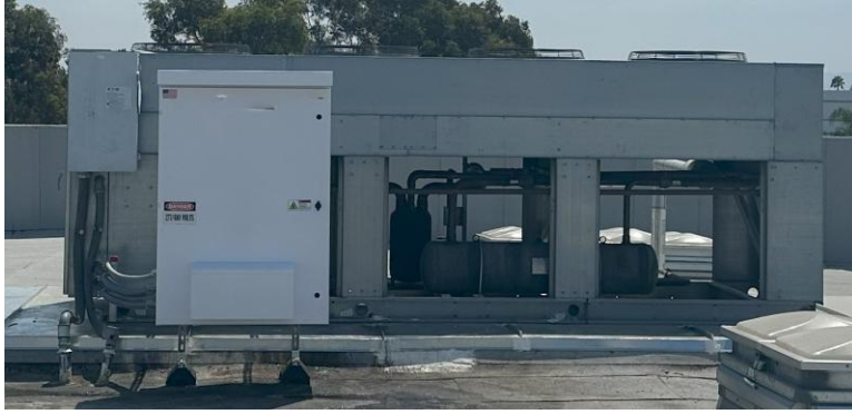
Figure 14: CU3 condensing unit with the ET.
