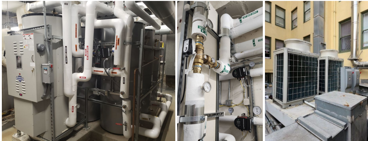
Figure 5: Swing tank and storage tank array, mixing valve, and rooftop HPWHs.
