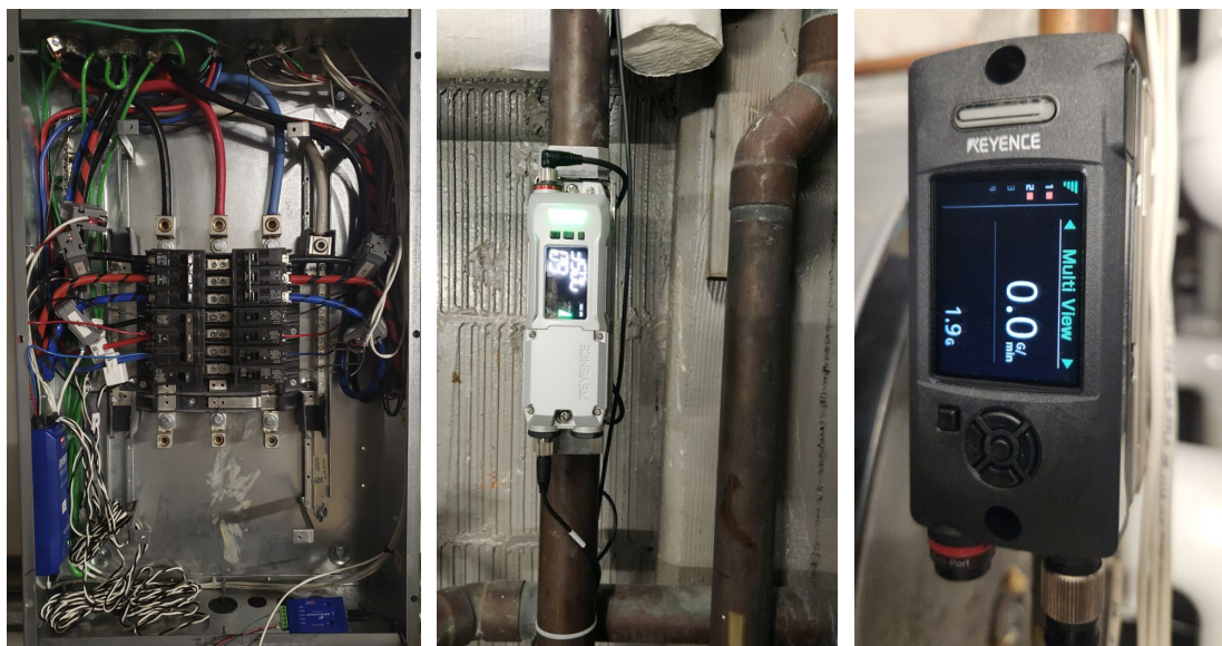
Figure 9: Swing tank power meter (P01), city water flowmeter (F01), and recirculation flowmeter (F02).
