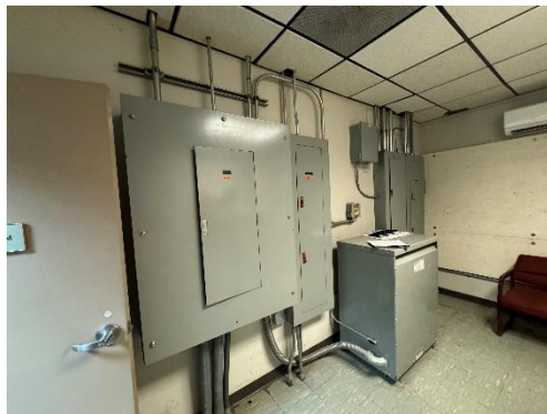
Figure C-32: Main Panelboard
