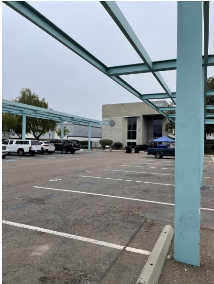
Figure C-1. Office Building Exterior.
