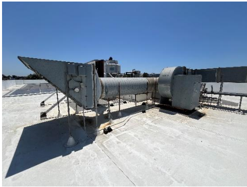
Figure C-6: Rooftop OA Supply Fan #1
