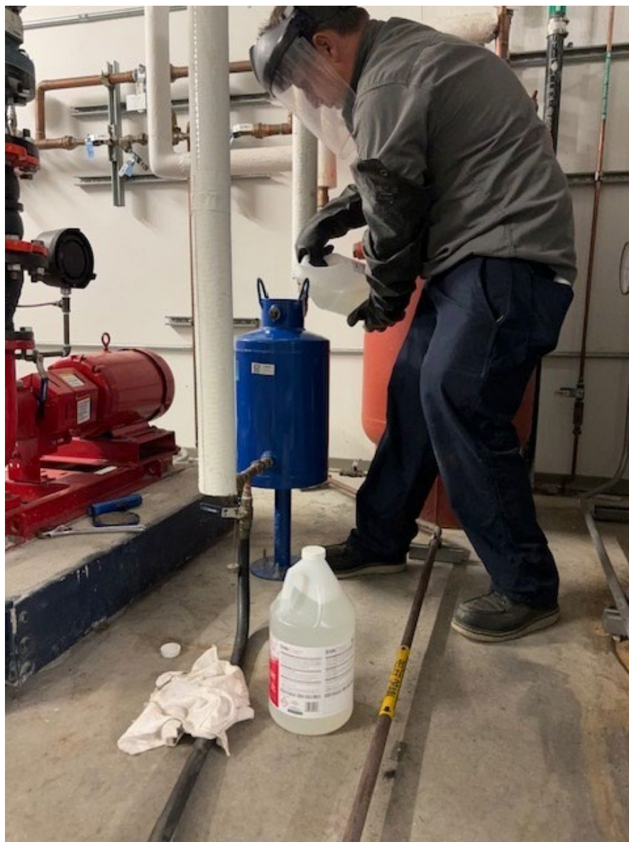
Figure 7: Installation of Hydronic Fluid Additive by qualified personnel at Site #1.
