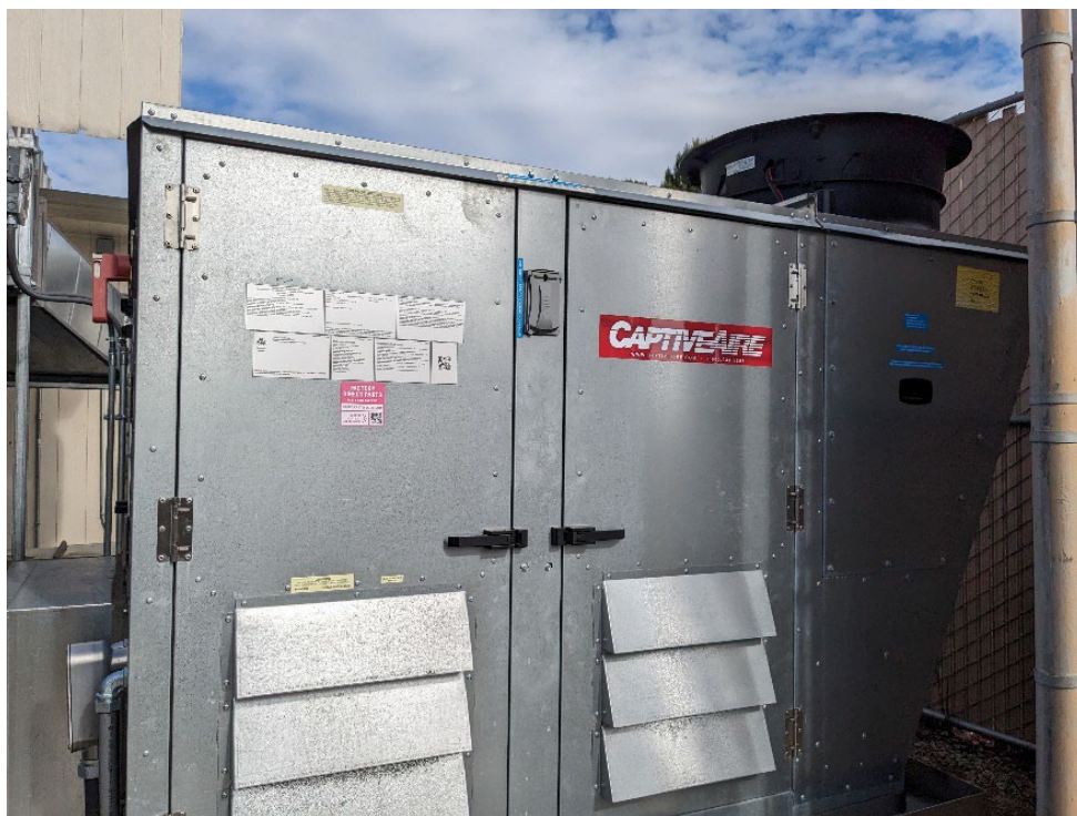
Figure 3: HP-2 at Site 1.
