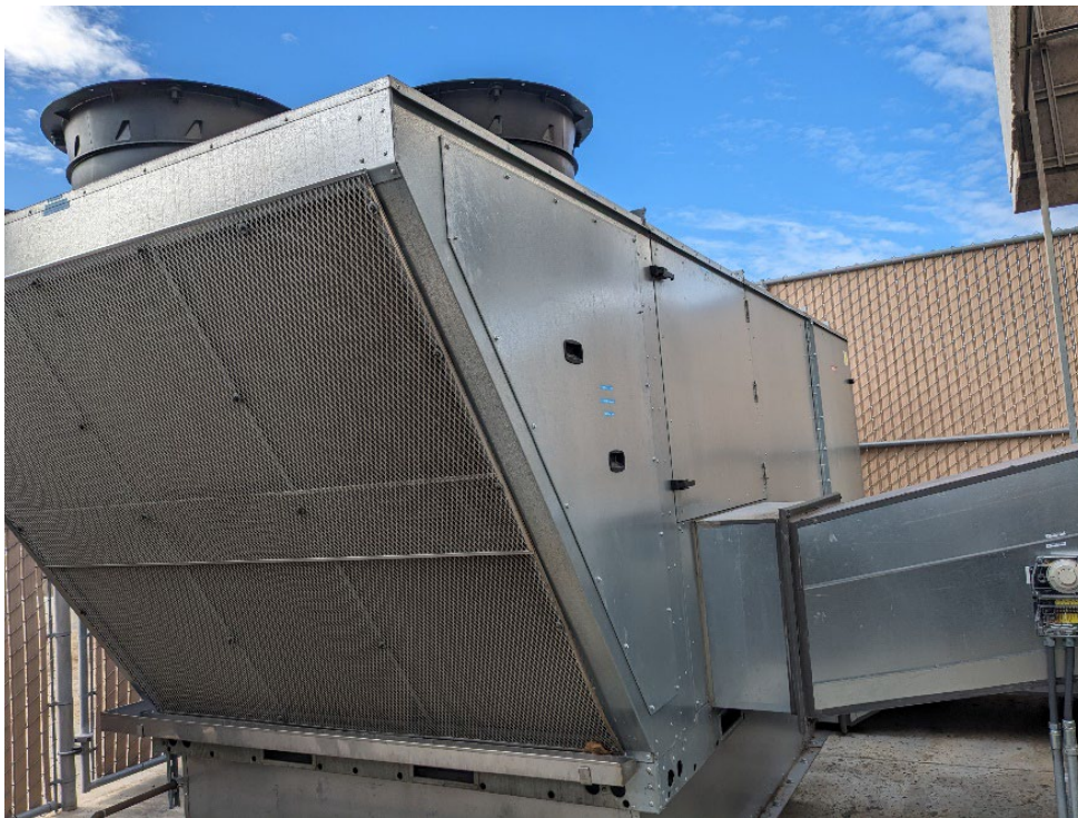
Figure 2: HP-1 at Site 1.
