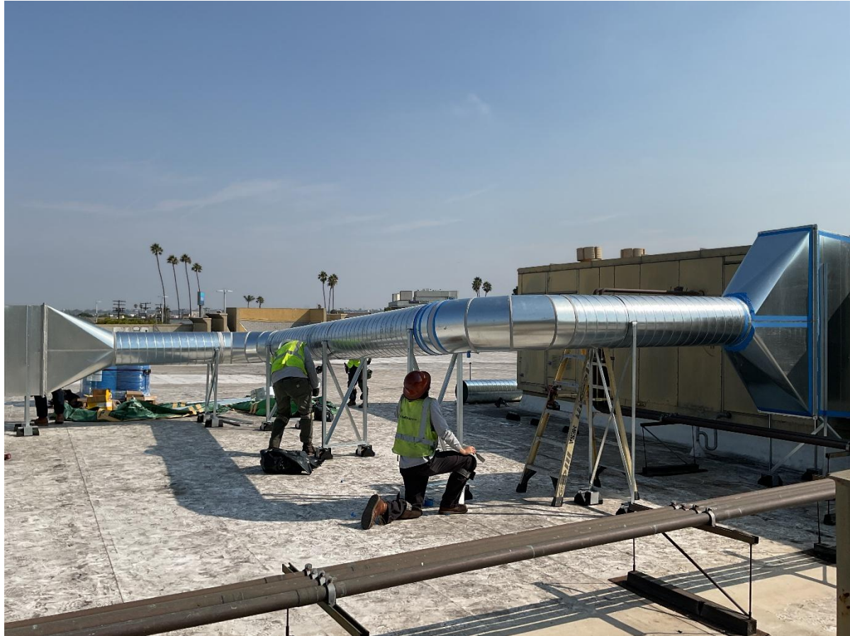
Figure 5: ES-LD-DOAS piping to existing rooftop air handler.
