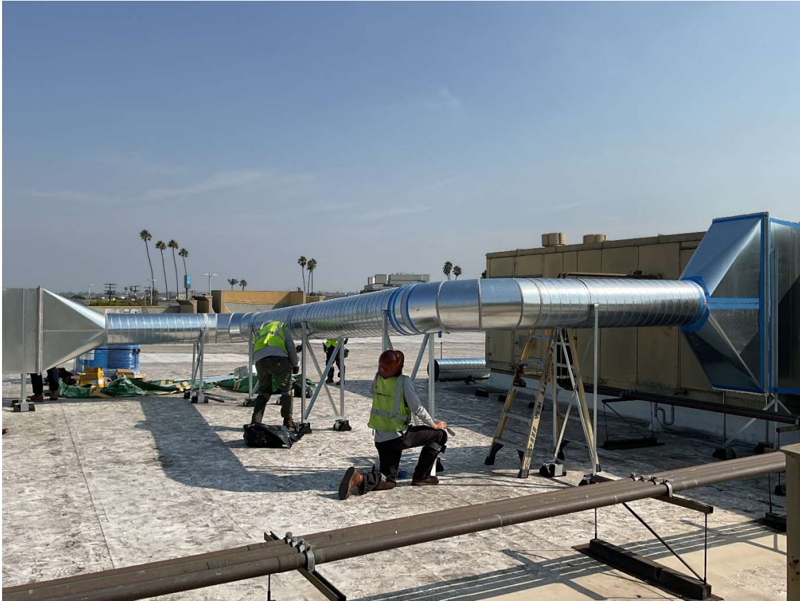
Figure 5: ES-LD-DOAS piping to existing rooftop air handler.
