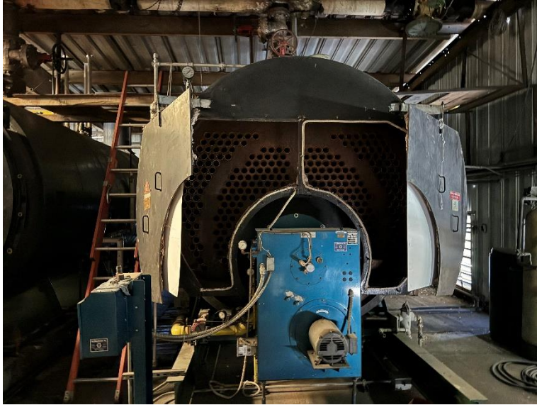
Figure 50: Greenhouse #3 steam boiler.
