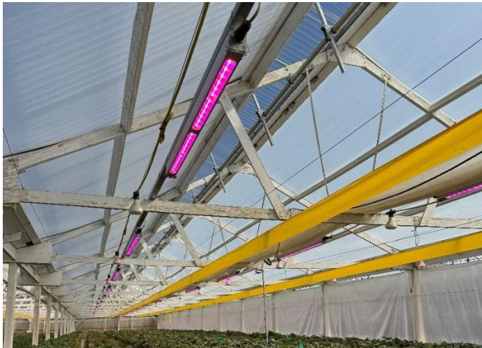
Figure 52: Greenhouse #3 strawberry zone supplemental lighting.
