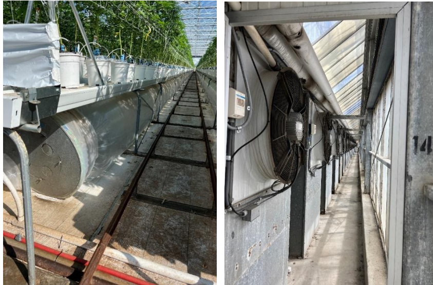
Figure 45: Duct socks and fans at Greenhouse #2.
