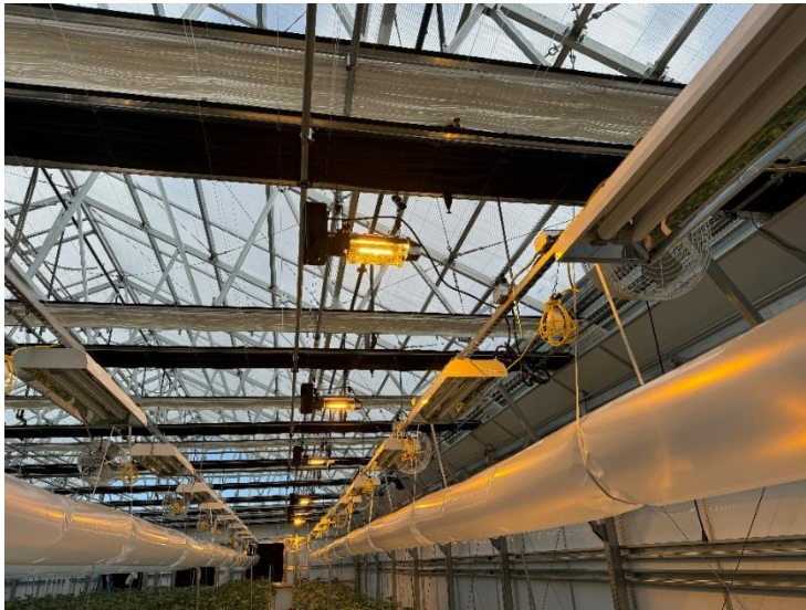
Figure 41: Greenhouse #1 typical flowering lighting zone.
