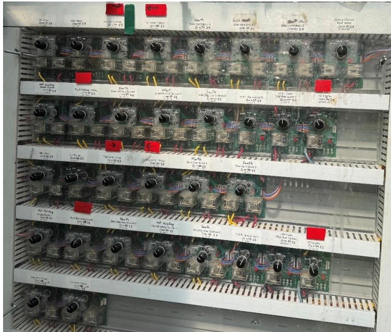
Figure 56: Integrated environmental controls serving Greenhouses L1 and L2.
