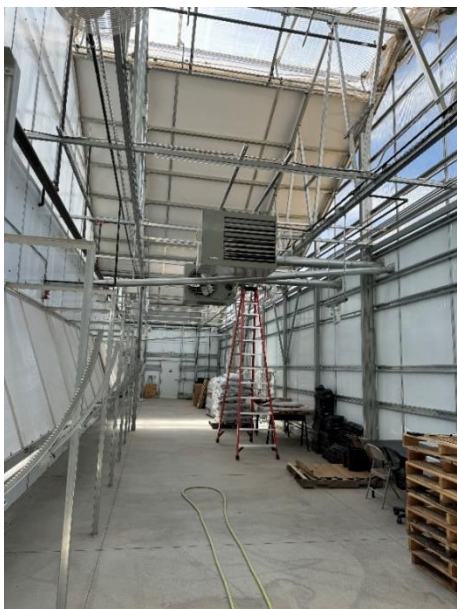
Figure 40: Greenhouse #1 head house heaters.
