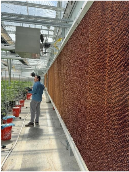
Figure 39: Greenhouse #1 wet wall.
