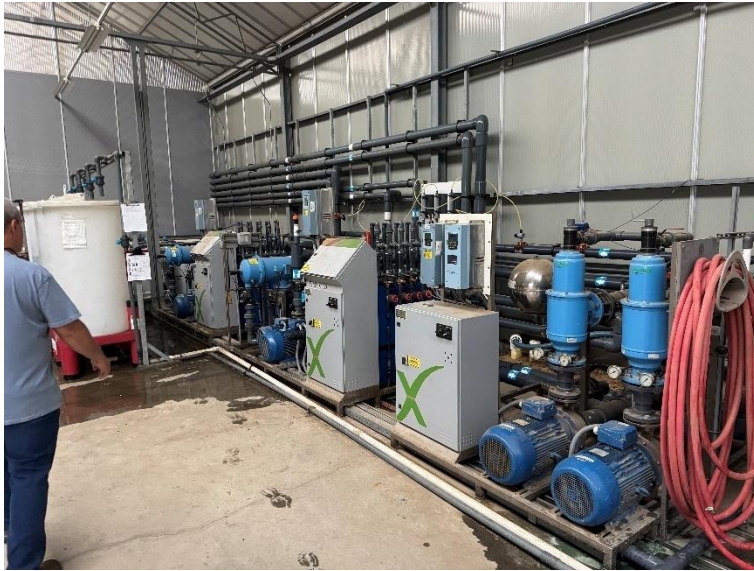
Figure 68: Irrigation and fertigation systems serving Greenhouse F.
