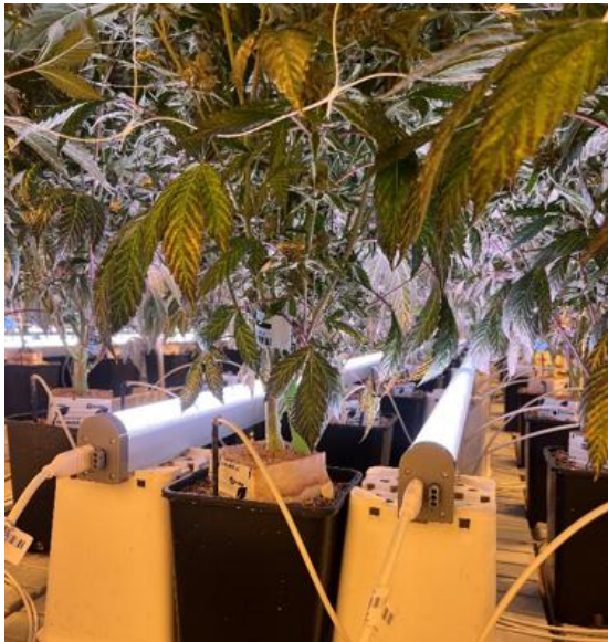
Figure 35: Under-canopy LED lighting at Indoor Farm #1.
