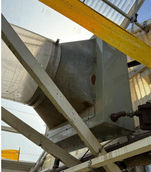
Figure 49: Greenhouse #3 steam fan coil.
