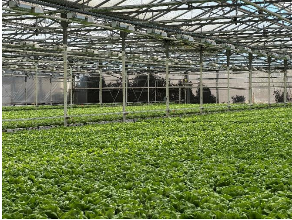
Figure 60: High-pressure sodium supplemental lighting serving Greenhouse L2.
