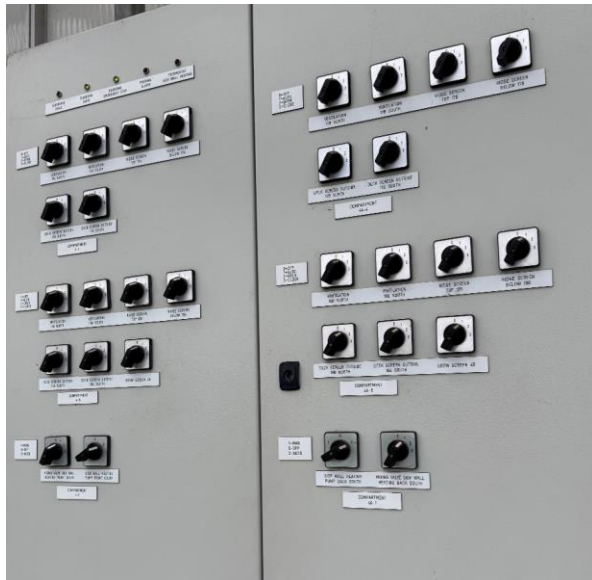
Figure 65: Integrated environmental controls serving Greenhouse F.
