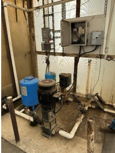
Figure 53: Irrigation pump skid.
