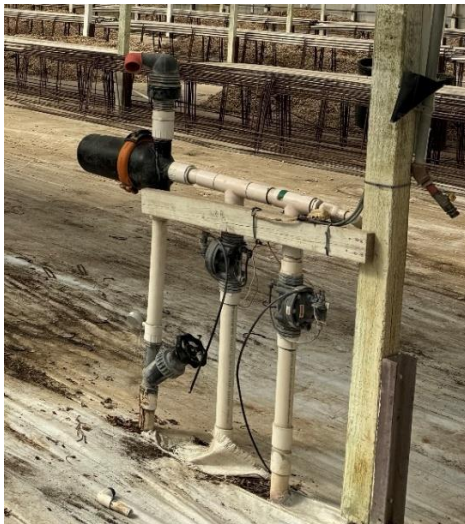
Figure 54: Irrigation valves.
