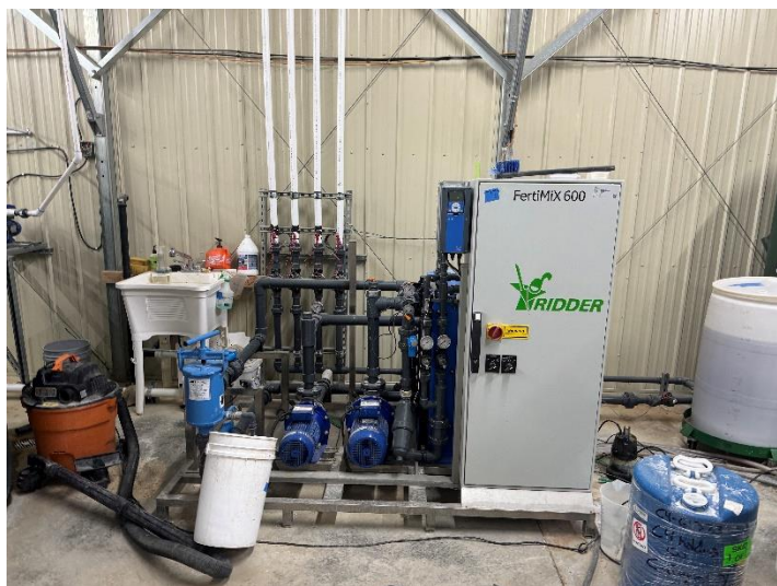
Figure 42: Greenhouse #1 irrigation pump and dosing skid.
