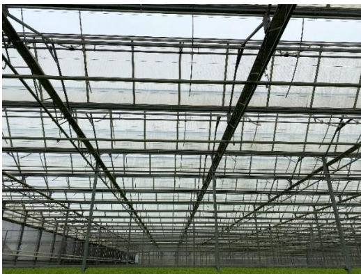
Figure 57: Greenhouse L1 curtain system.
