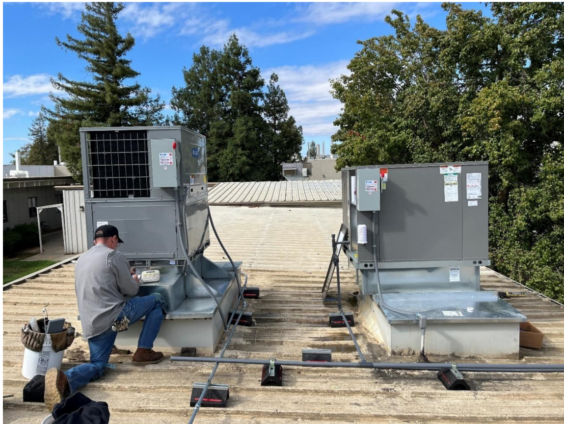
Figure 8. Heat pump RTUs photographed during installation
