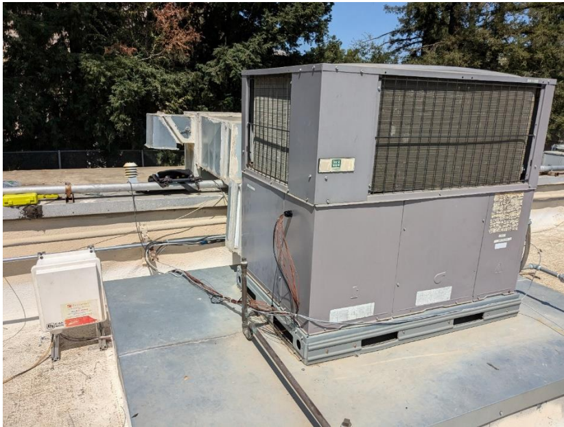
Figure 5. Gas-fired RTU and data acquisition enclosure for temperature, humidity, pressure, and component
