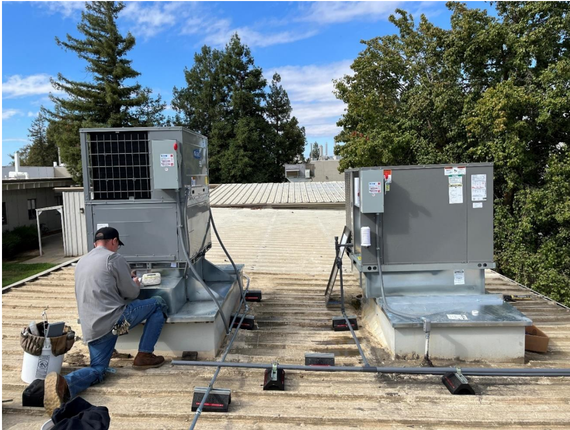
Figure 8. Heat pump RTUs photographed during installation
