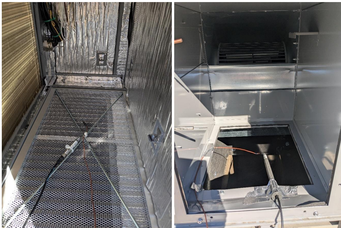
Figure 10: Return (left) and supply (right) temperature and humidity probes.
