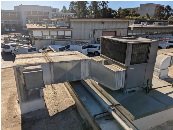
Figure 2. Photo of existing gas-fired RTU used as a baseline for comparison
