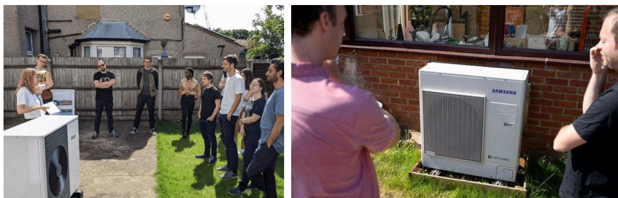
Figure 14. Visitors on a home tour learning about heat pumps
