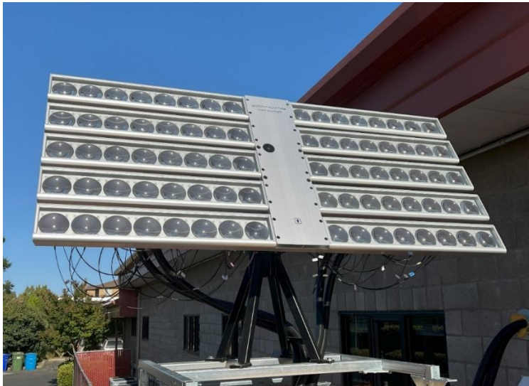
Figure 1: STF fiber optic daylighting system, fully installed.
