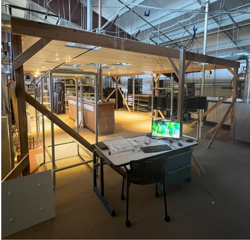
Figure 6: STF demonstration space under construction.
