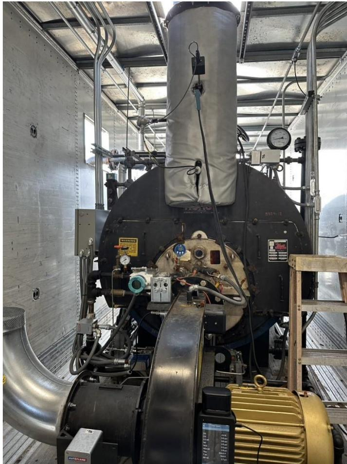
This boiler burner using the ClearSign Core technology has exceptional flexibility for controlling NOx emissions. During the site visit, we were able to tweak the burner to operate close to sub 1 ppm NOx. From conversations with representatives, they claimed that they have not yet even come close to “optimizing” the burner.
