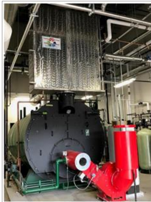
Figure 25: Economizer- Two stage stacked (manufacturer C) [18]
