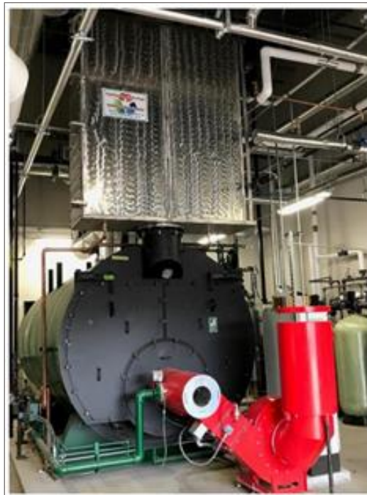
Figure 25: Economizer- Two stage stacked (manufacturer C) [18]
