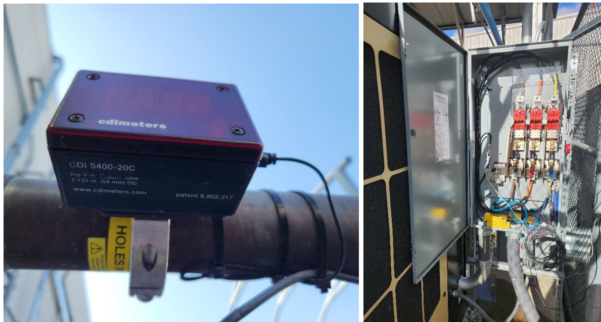
Figure 7: Air compressor supply airflow and pressure meter and power metering.
