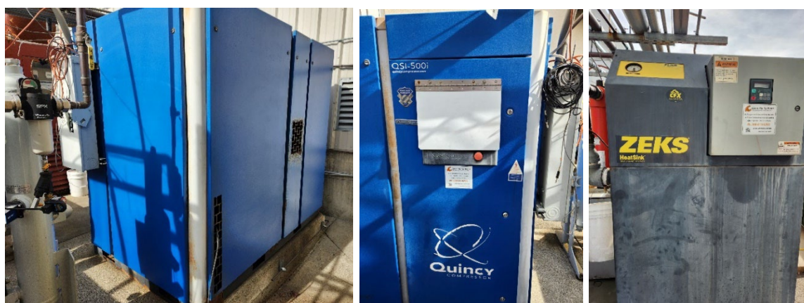
Figure 5: Lag air compressor (Quincy QSi-500i) and dryer.
