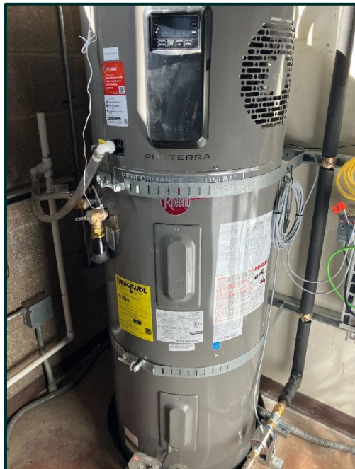
Figure 11. Rheem Wi-Fi-enabled heat pump water heater (left) and unit communication diagram (right).
