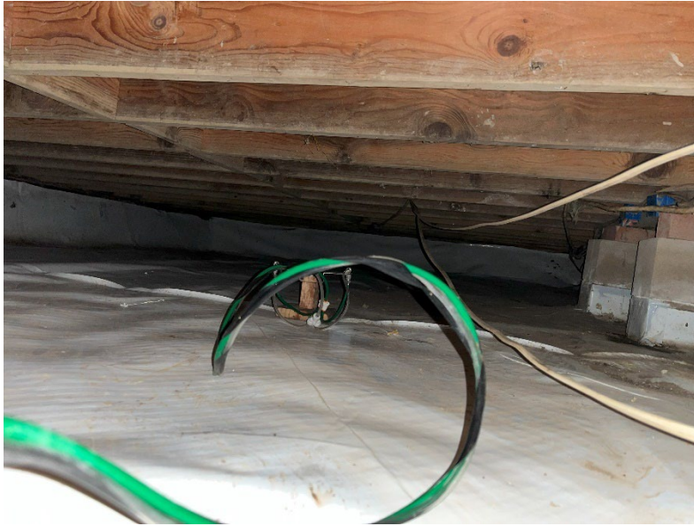
Figure 6. Photo of crawlspace sealed at Site 4.
