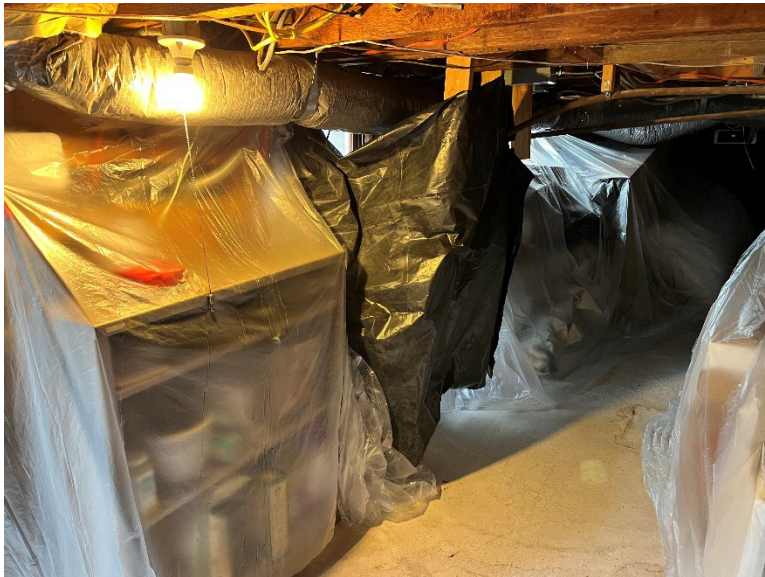
Figure 4. Example of plastic used to protect a storage area.
