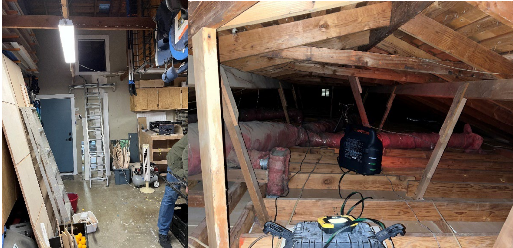
Figure 8. Attic access hole (left) and view from inside the attic (right).
