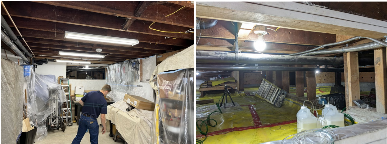
Figure 2. Basement/crawlspace area of Site 1.
