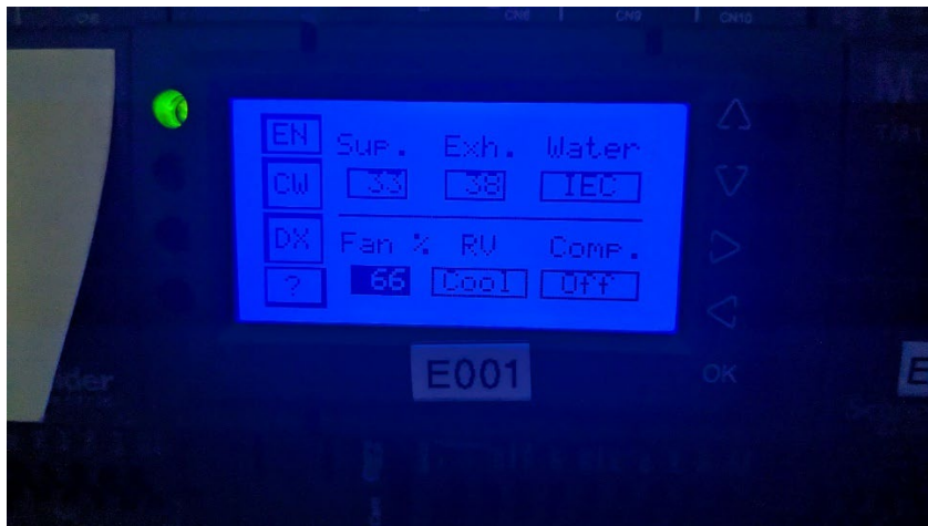
Figure 10. Control interface for Hybrid RTU.
