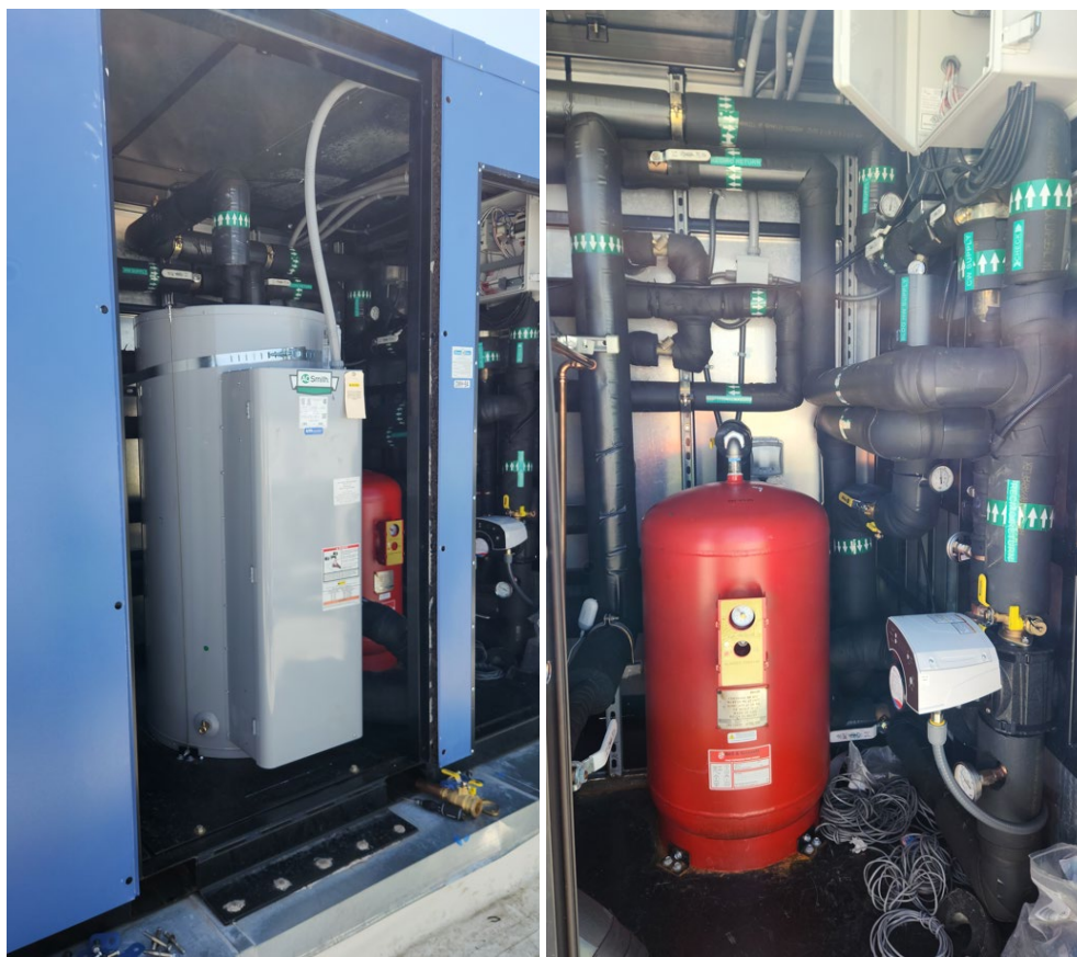
Figure 5: Swing tank and plumbing located inside packaged unit.
