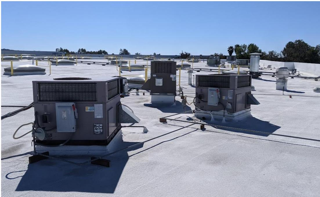
**Figure 11: Packaged rooftop air conditioners at Site 1**
