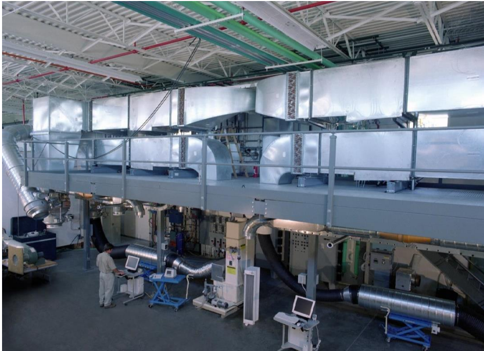
Figure 8. NREL Advanced HVAC Systems Lab, Thermal Test Facility
