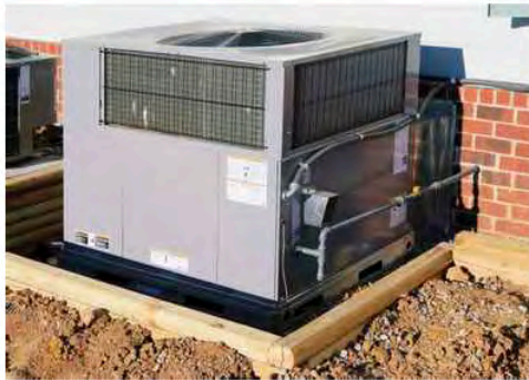
Packaged Gas Furnace Air Conditioner [i.e. Dual Pack] (ducted)
