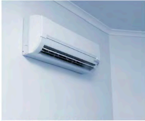
Mini Split Air Conditioner / Heat Pump (ductless)
