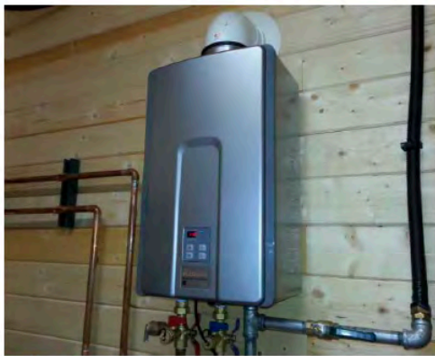
Tankless - Gas water heater
