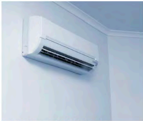
Mini Split Air Conditioner / Heat Pump (ductless)
