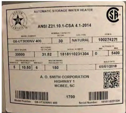
Storage Tank - Gas water heater nameplate
