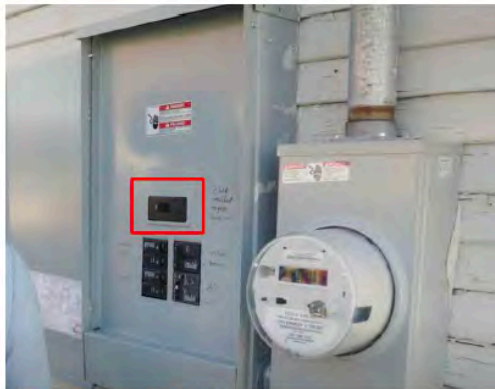
Main breaker next to electrical meter
