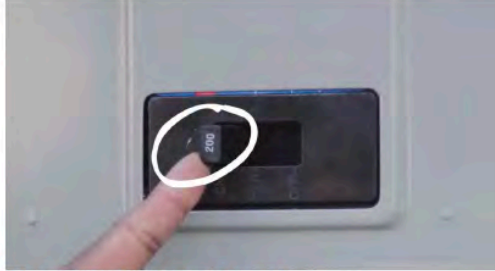
'Main circuit breaker' or 'main breaker'
