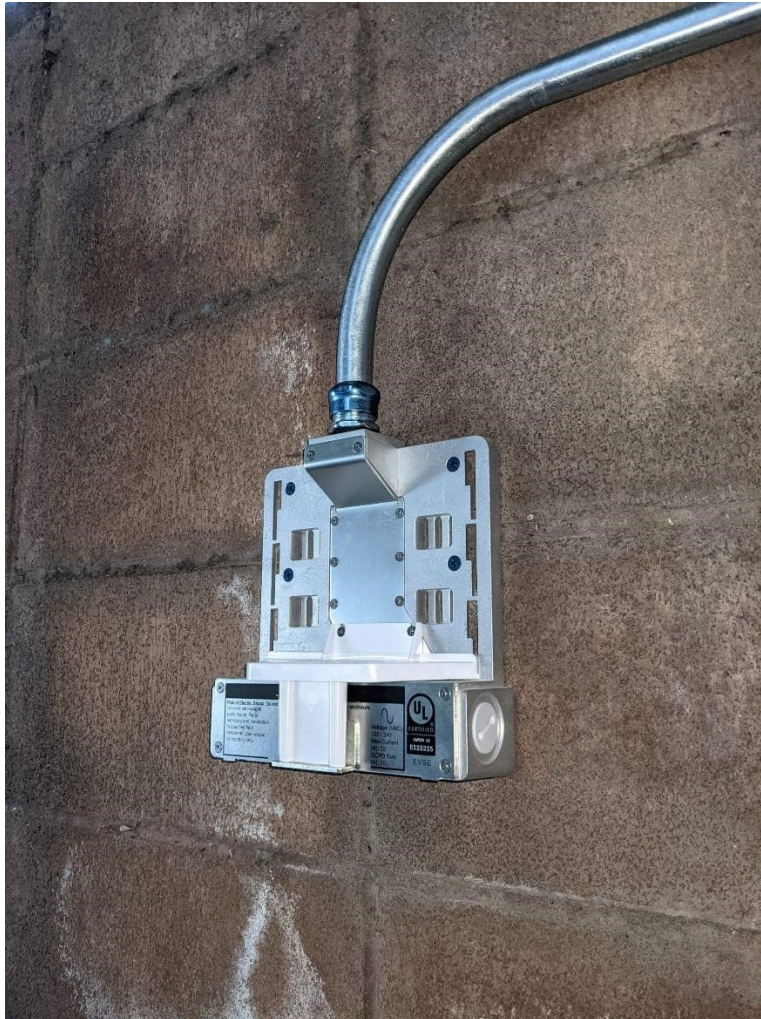
Figure 18: Charging Base Installed at Site 1
