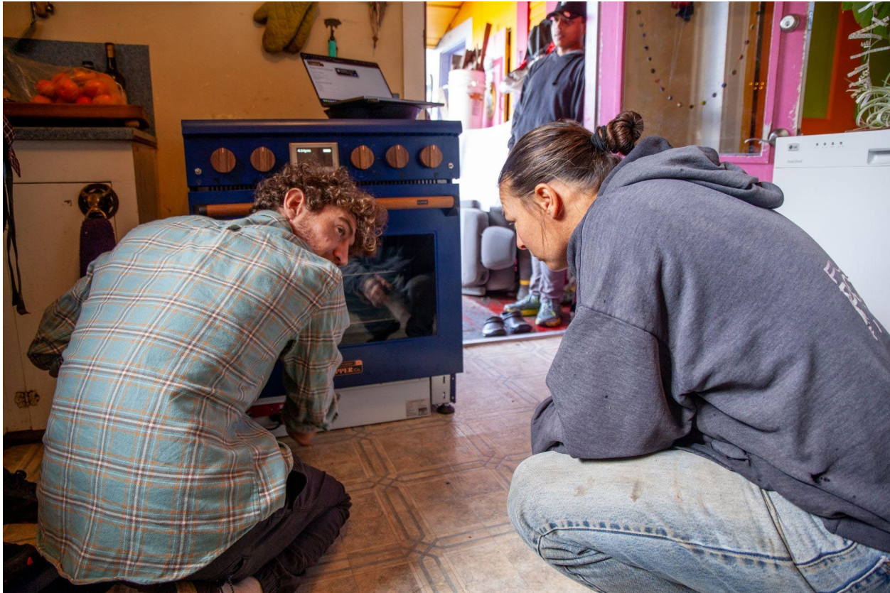
Figure 27: Prototype unit being installed at Redwood Energy Home Base.
